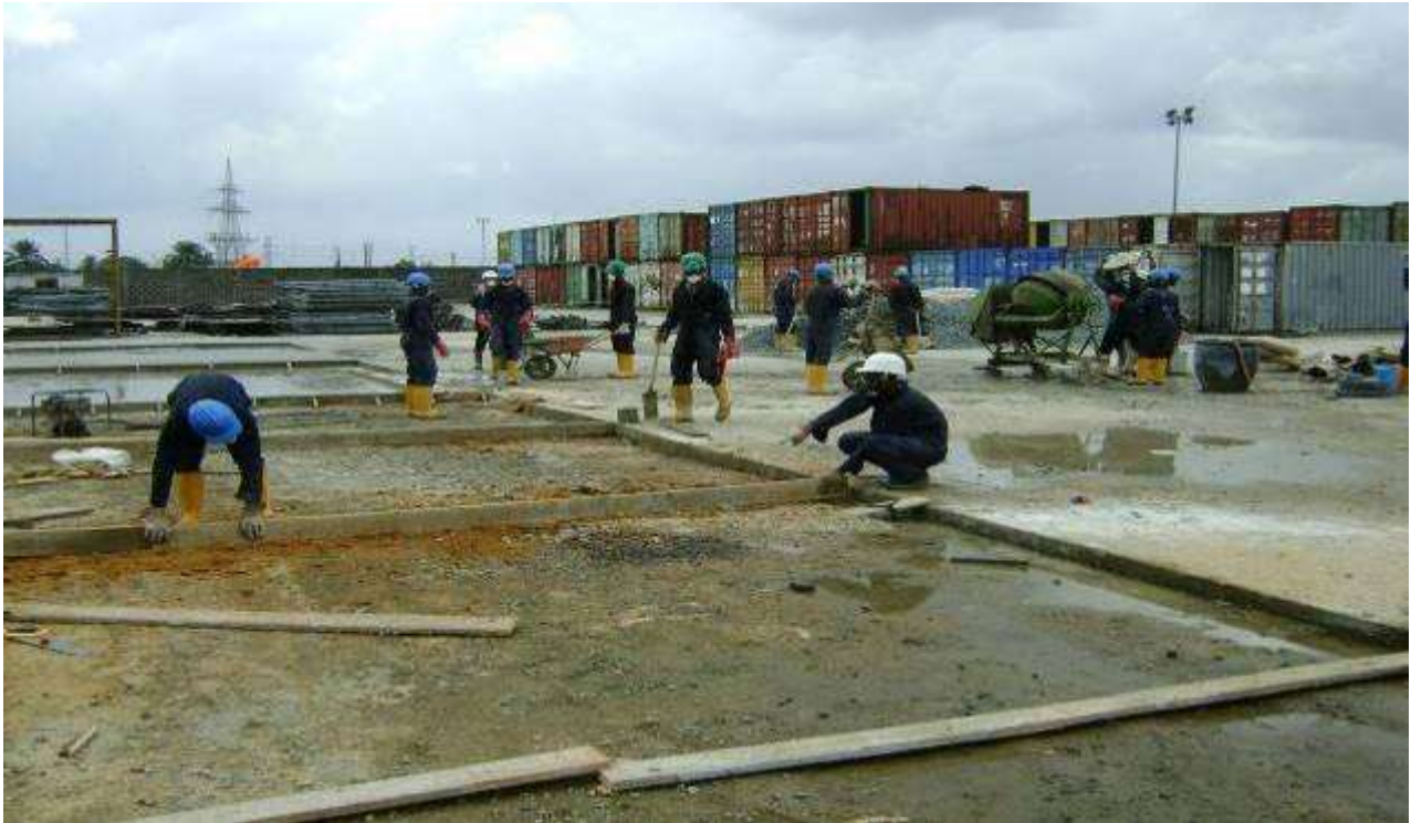
Construction of form work & ground preparation and concrete casting in progress on the concrete hard stand construction at S.P.D.C Industrial Area - East by Lumkalt Energy Limited.
