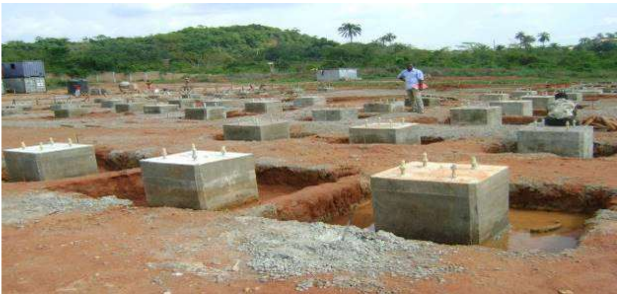
Placement of Anchors & Reinforcement and concrete works on equipment foundations at New Abeokuta 132/33Kv Substation and 132Kv DC Transmission lines.
