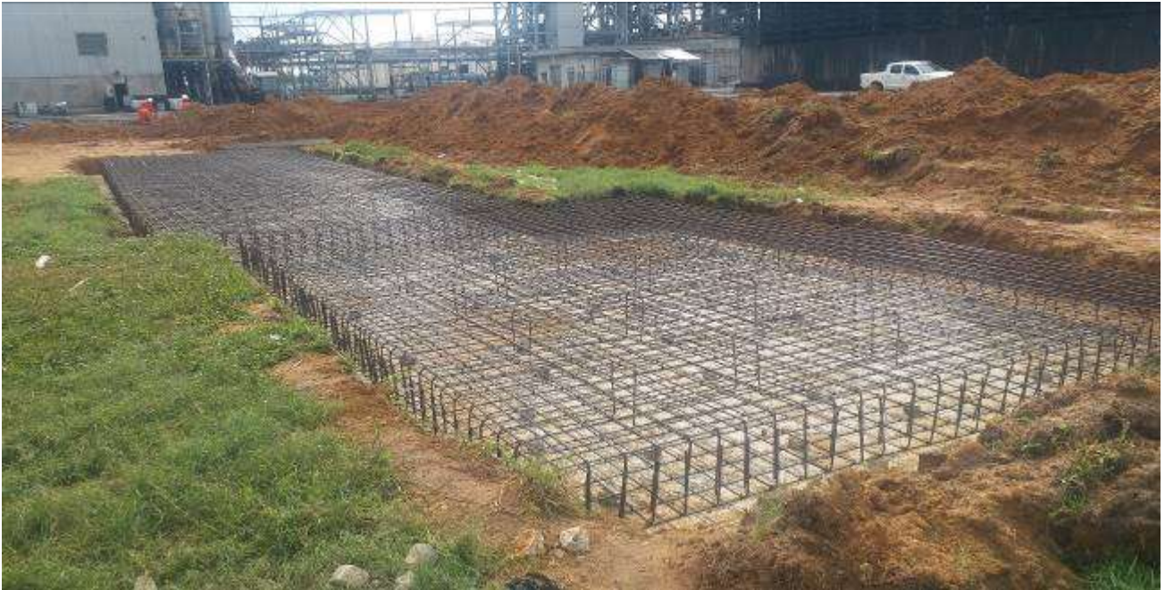
Reinforcement Work ongoing at Notore gas turbine power plant- By Lumkalt Energy Limited .
