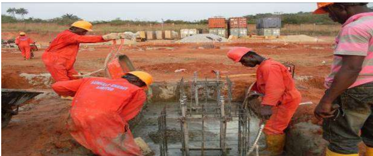
Technical discussion at site between Client's Project Manager & Sub-contractor's MD. Concrete works also ongoing in the equipment foundation at New Abaokuta.
