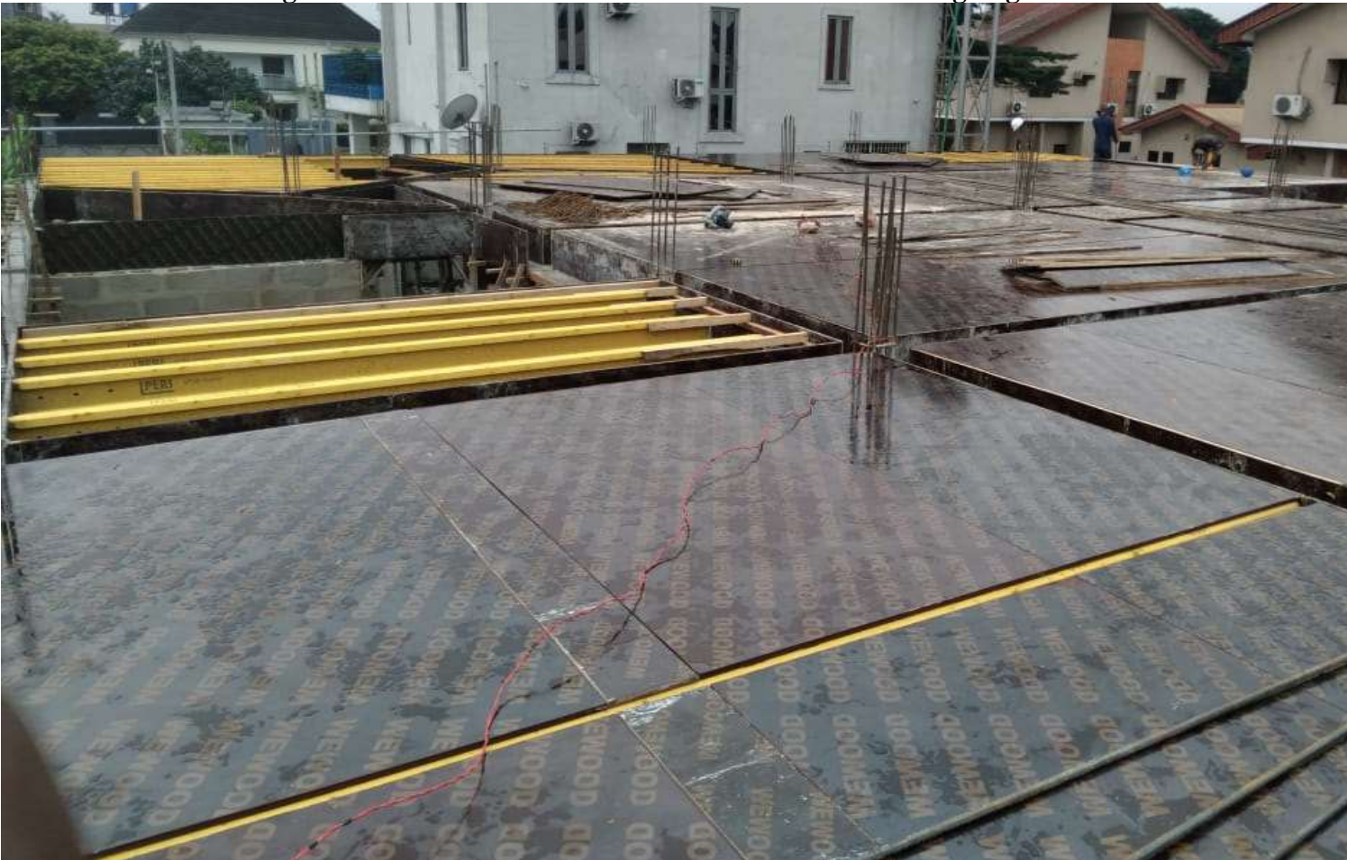
Progress work on first floor beams and slab formwork Ongoing
