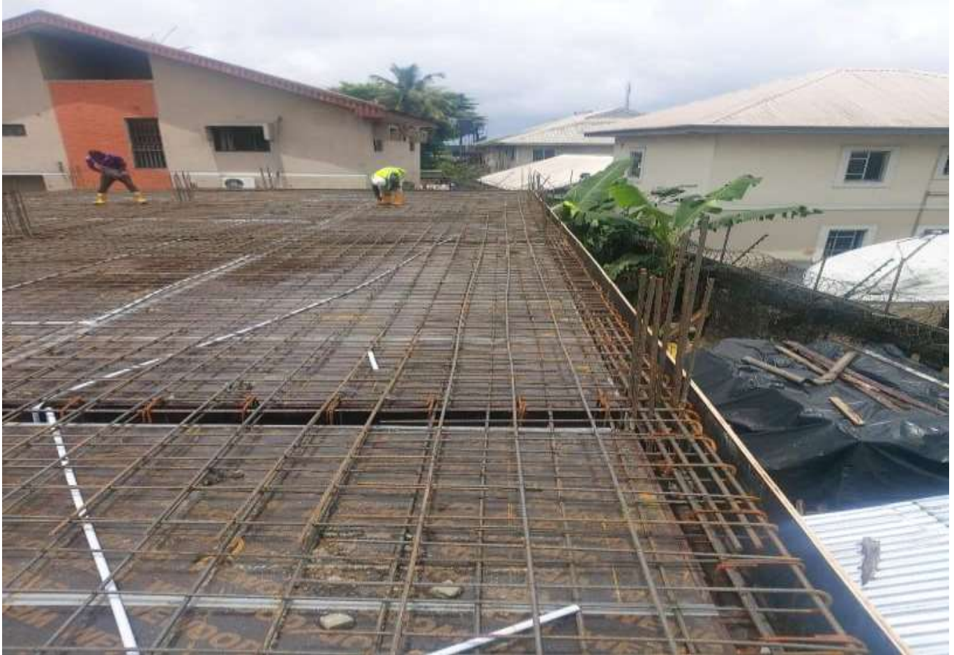
Placement & setting of first floor Reinforcement, Electrical & Mechanical pipework Ongoing
