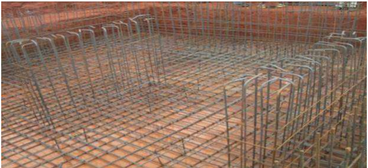
Layers of hardcores been layed on the excavated floor, Concrete Blinding of floor completed and Reinforcement Placed in the transformer foundation - Lumkalt Energy Limited
