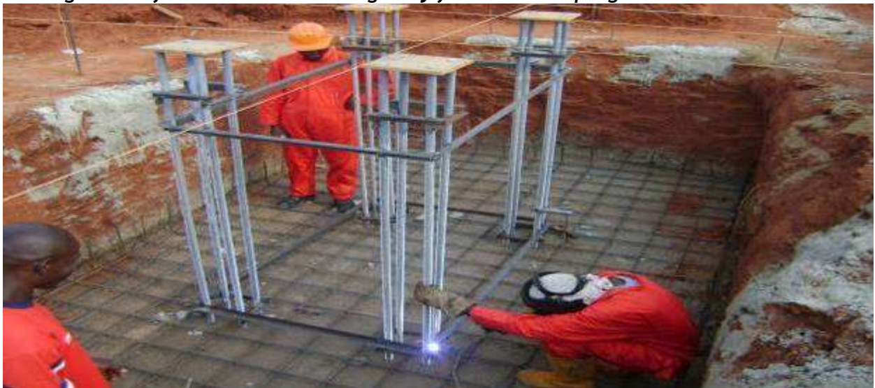
Welding of anchors bolt in position in progress during gantry foundation construction at New Abeokuta.
