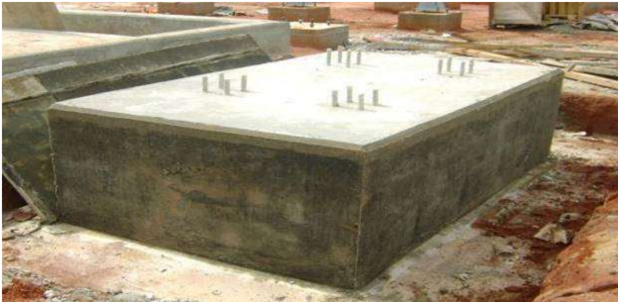
Completed Gantry foundation ready for side backfilling & compaction at New Abeokuta.
