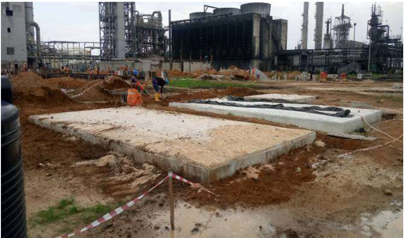
Equipment foundation concrete works completed at Notore gas turbine power plant- By Lumkalt Energy Limited .
