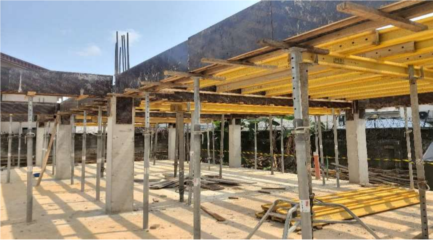
Progress work on first floor beams and slab formwork Ongoing
