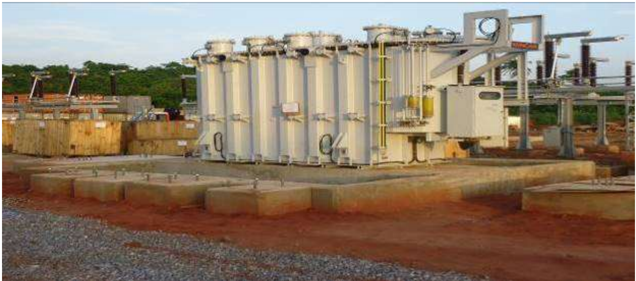
Transformer foundation completed and 60MV Transformer Erected.- Lumkalt Energy Limited
