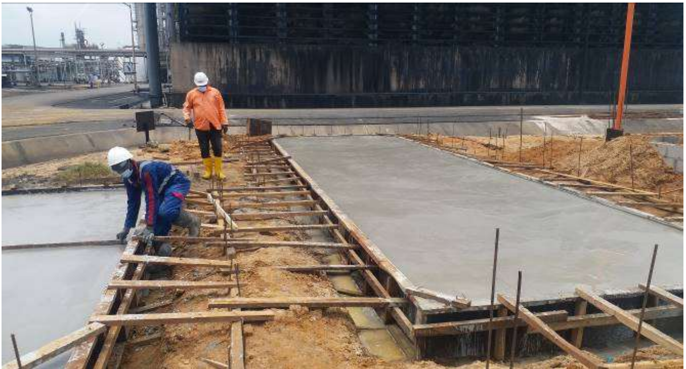
Equipment foundation concrete works completed at Notore gas turbine power plant by Lumkalt Energy Limited .
