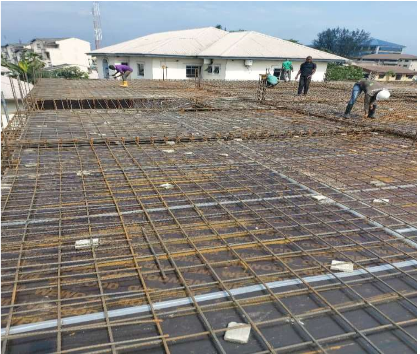
Placement & Setting of First Floor to Second Floor Reinforcement, Edge Formwork, Electrical & Mechanical pipework Ongoing
