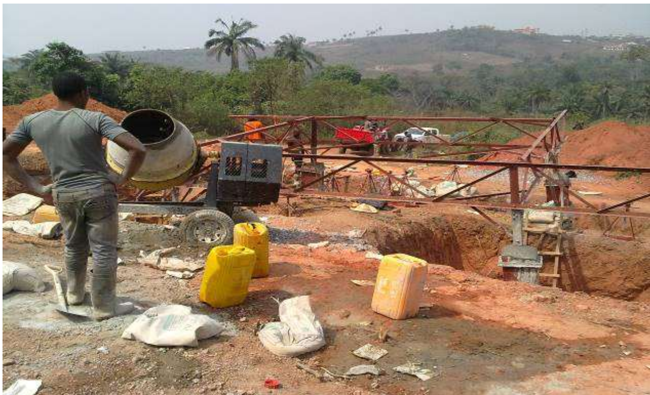
Casting of Chimney completed and ready for formwork removal and Backfilling (New Abeokuta to Papalanto) - by Lumkalt Energy Limited
