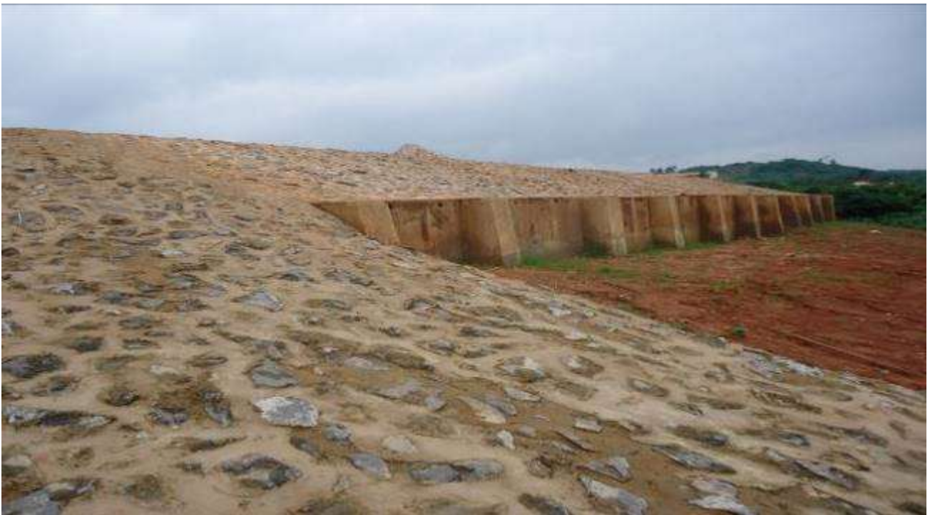
Completed Retaining Wall with all Inclinations Stoned Pitched to Finish at New Abeokuta.
