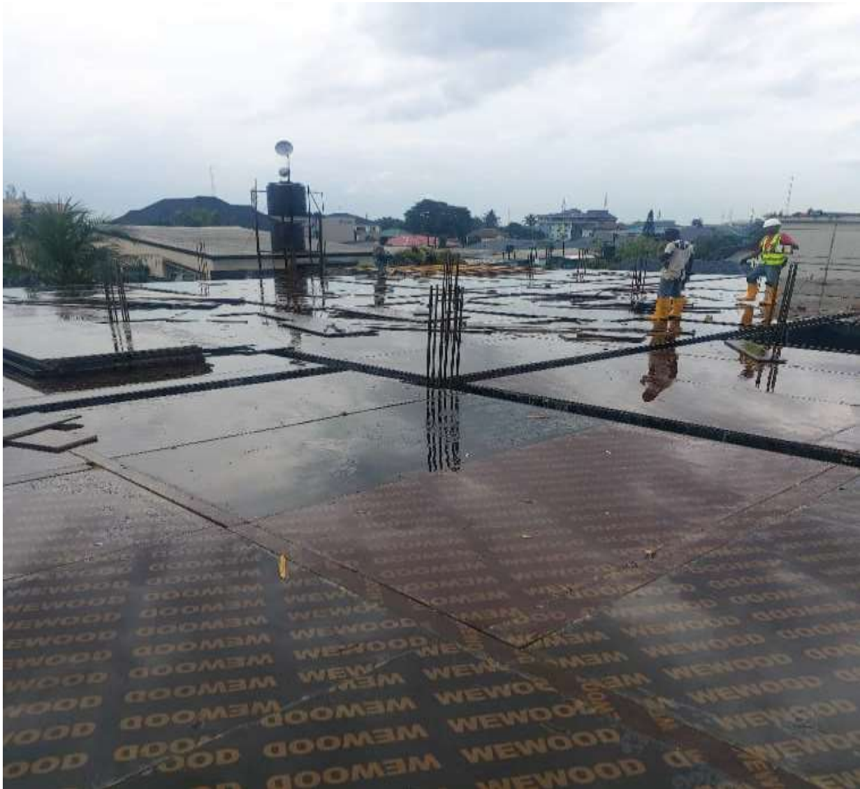
Placement of second floor beam and slab formwork Completed
