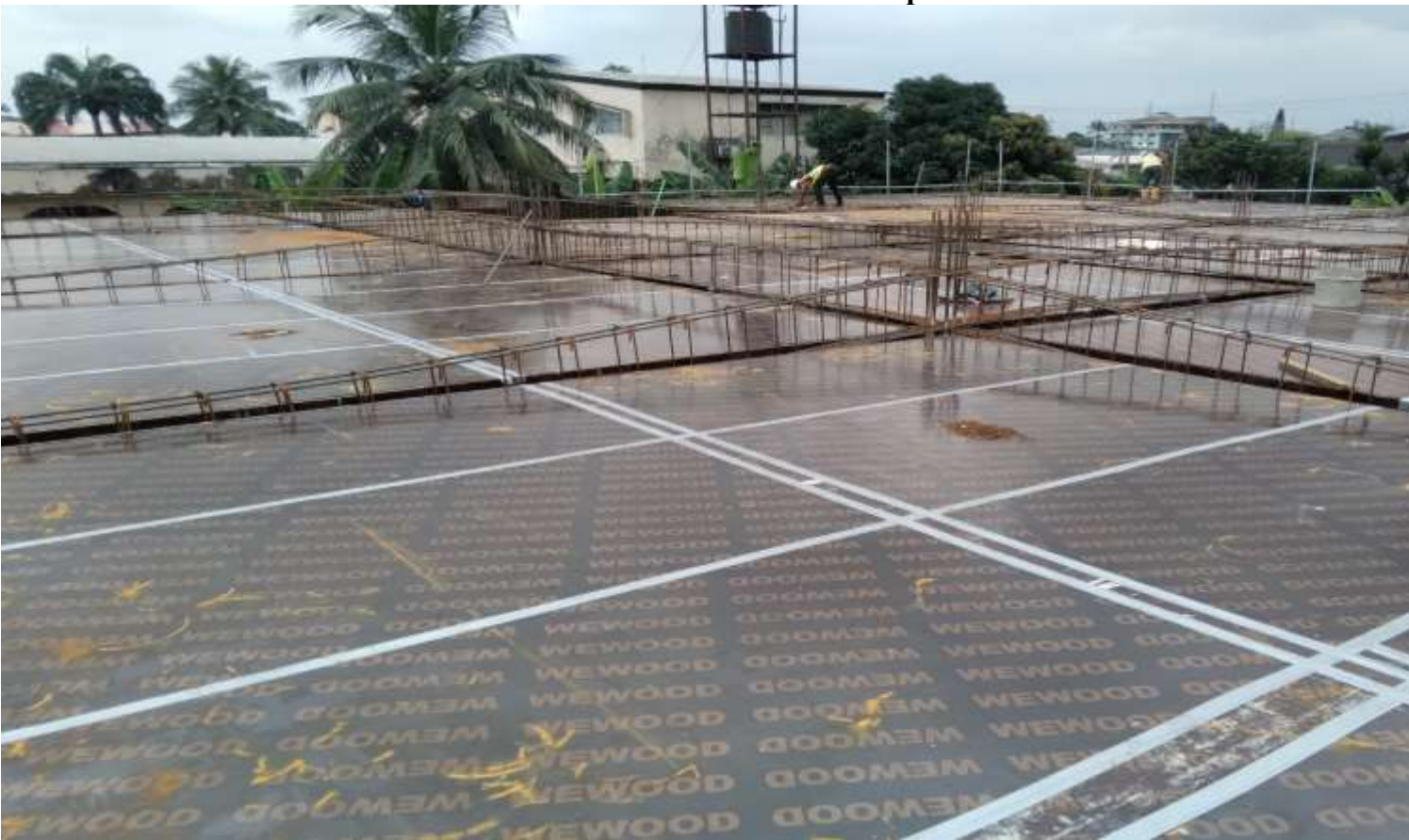
Placement & setting of first floor Beams Reinforcement Ongoing
