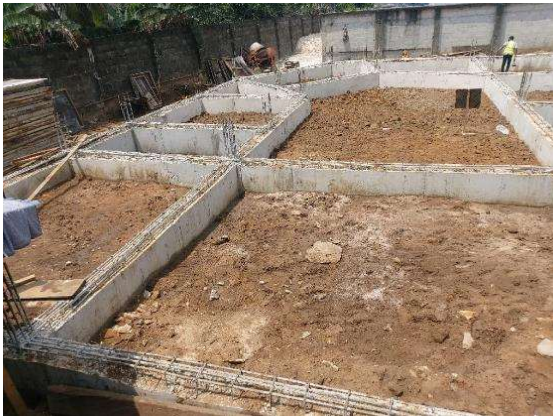
Ground beam concrete works completed at Principles Law Partnership, GRA Phase II, Port Harcourt, Rivers State -By Lumkalt Energy Limited .
