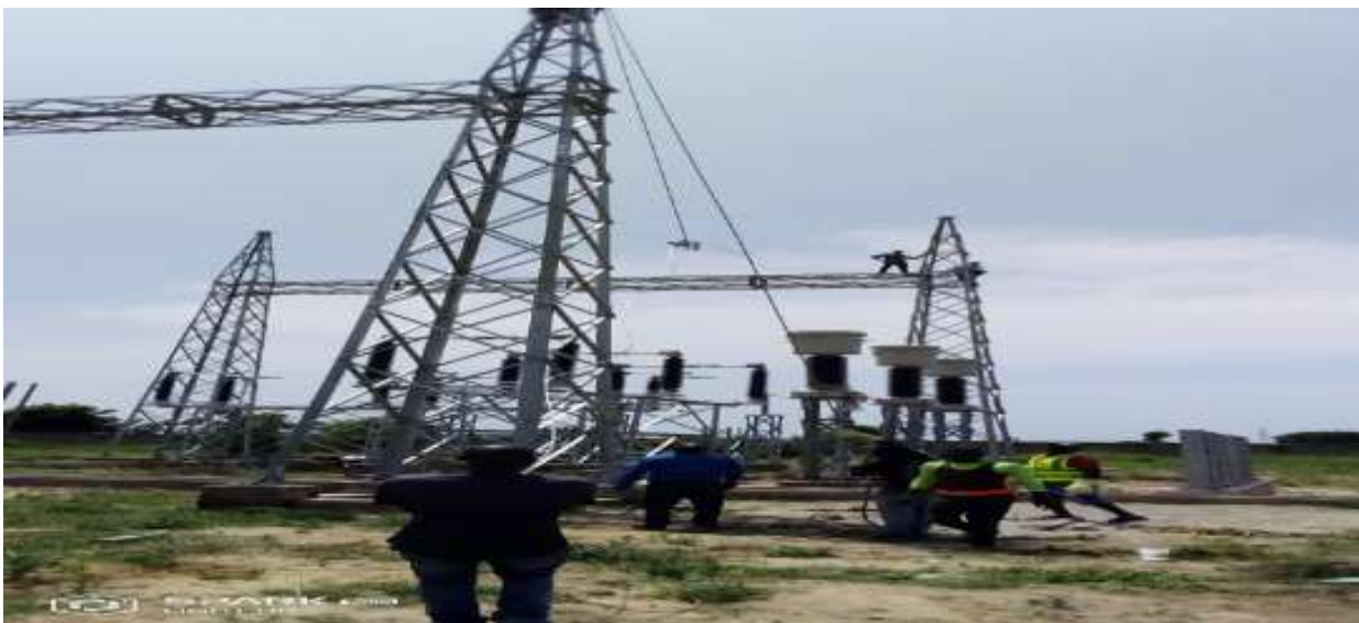
Completed Erection/Electromechanical works at 132/33Kv Substation - Gagarawa in Jigawa State. By Lumkalt Energy Ltd / Katamegos Africa Ltd.
