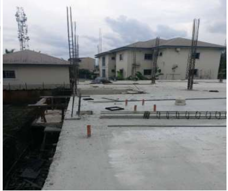
Placement of First Floor to Second Floor Column Reinforcement Ongoing
