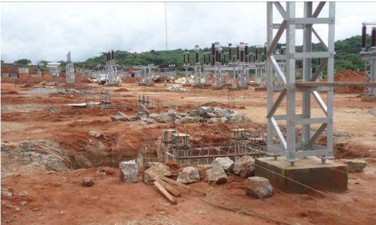
Foundations alignment checks by Engineers ongoing, Equipment installation on foundations ongoing and Gantries foundation construction in progress at New Abeokuta by - Lumkalt Energy Limited.
