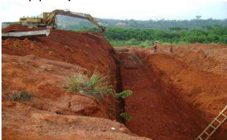
Mechanical Excavation work in progress for a massive reinforced concrete retaining wall at New Abeokuta.
