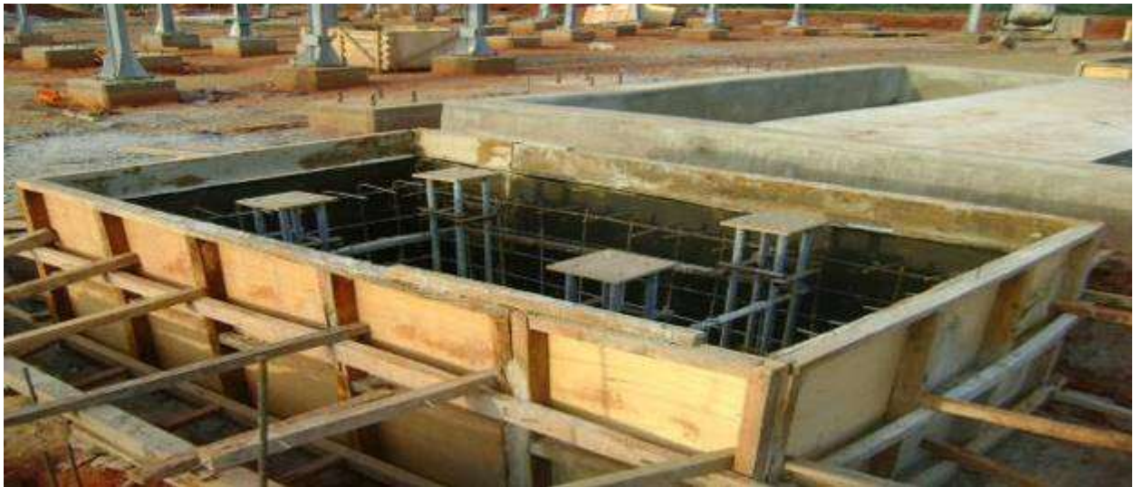
Completed form work for gantry foundation ready to receive concrete at New Abeokuta.
