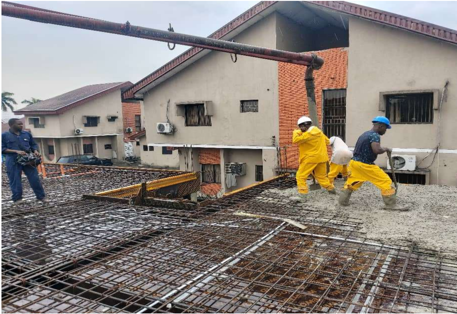
Concrete placement of the first floor slab and beam ongoing
