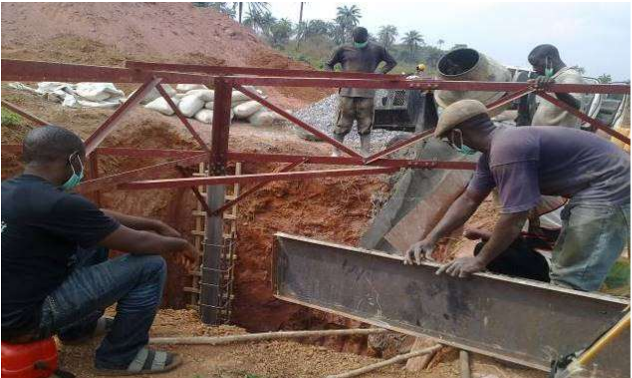
Installation of Template to the chimney and pads (New Abeokuta to Papalanto) - by Lumkalt Energy Limited
