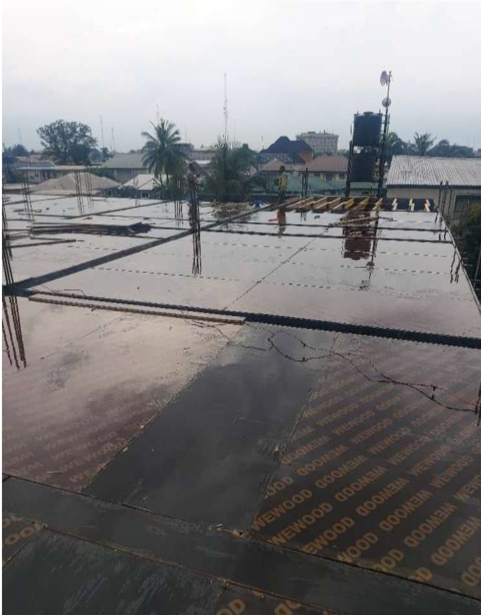
Placement of second floor beam and slab formwork Ongoing
