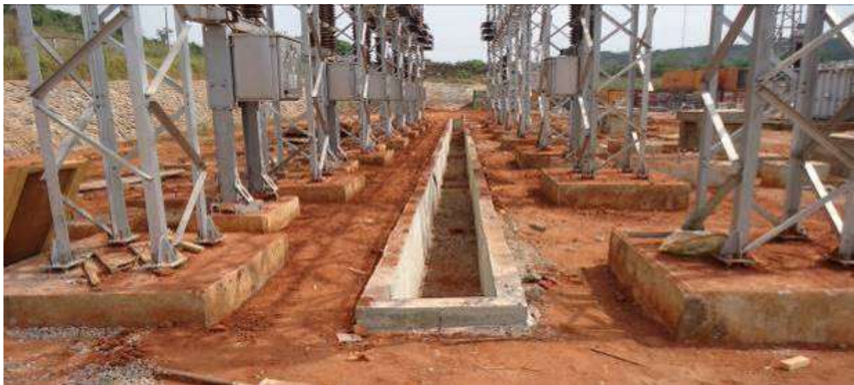
Completed 33kv Equipment foundations and cable trench at New Abeokuta SS.
