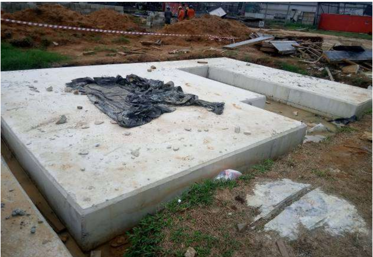
Equipment foundation concrete works completed at Notore gas turbine power plant By Lumkalt Energy Limited .
