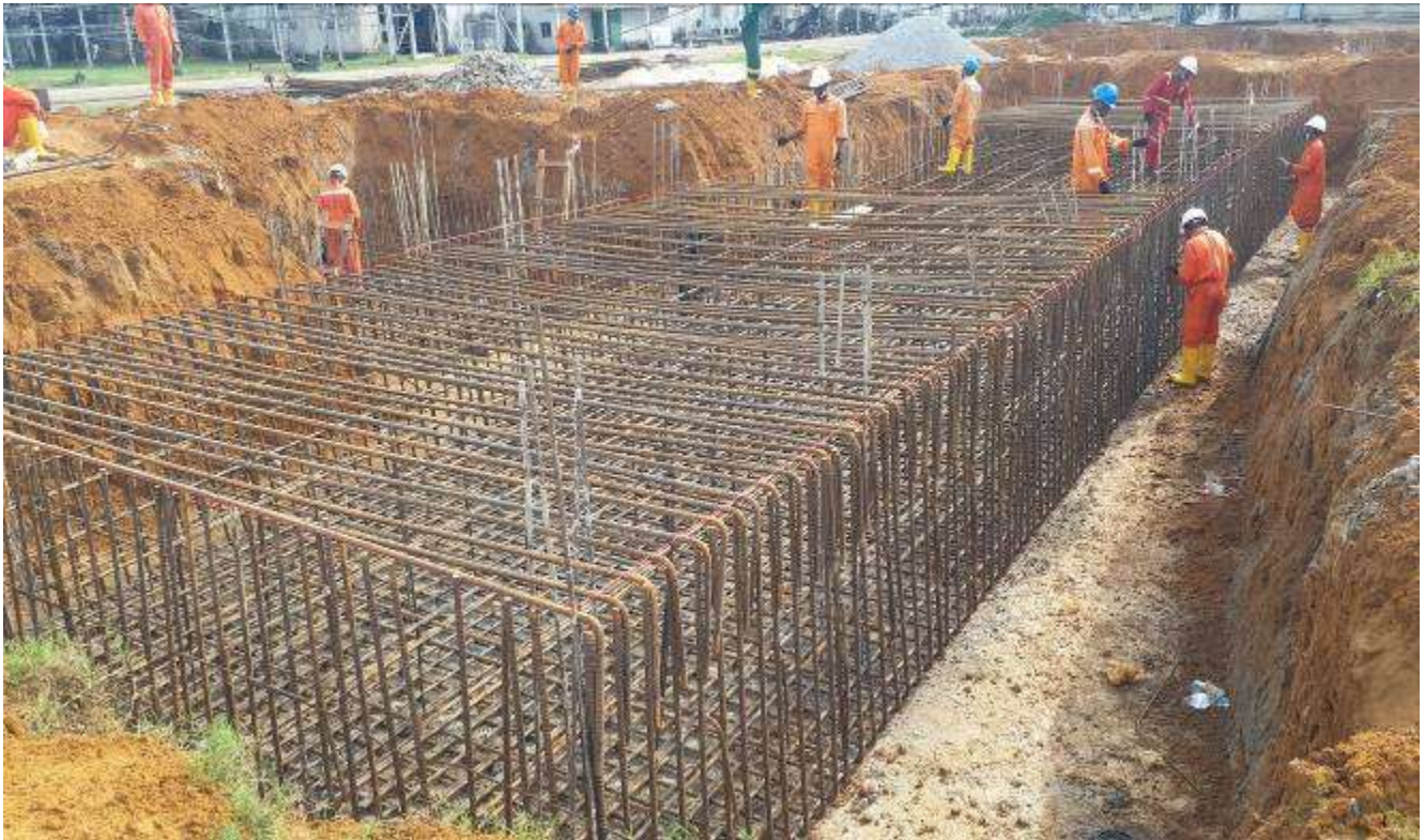
Reinforcement Work ongoing at Notore gas turbine power plant- By Lumkalt Energy Limited .
