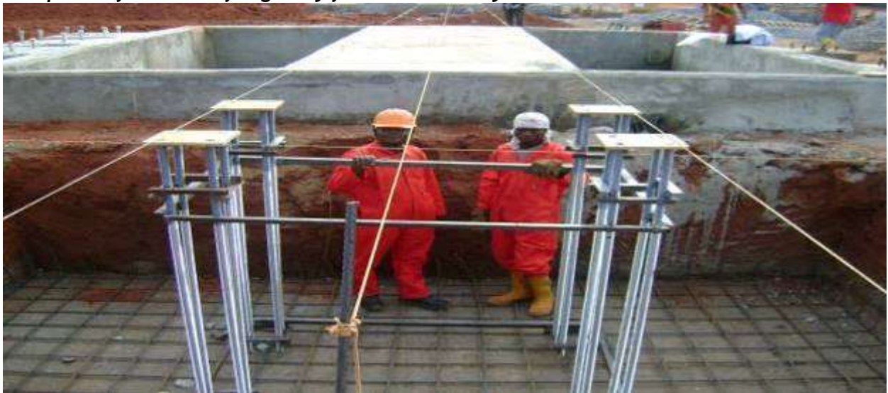
Alignment of Anchors bolts in the gantry foundation in progress at New Abeokuta.
