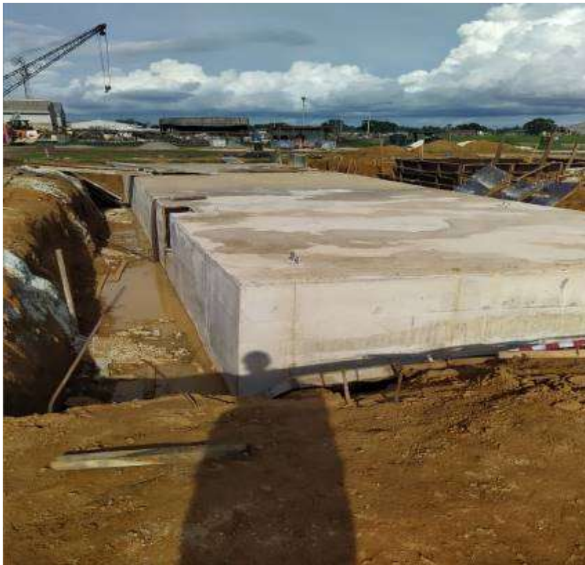
Gas turbine foundation concrete work completed at Notore gas turbine power plant - By Lumkalt Energy Limited.
