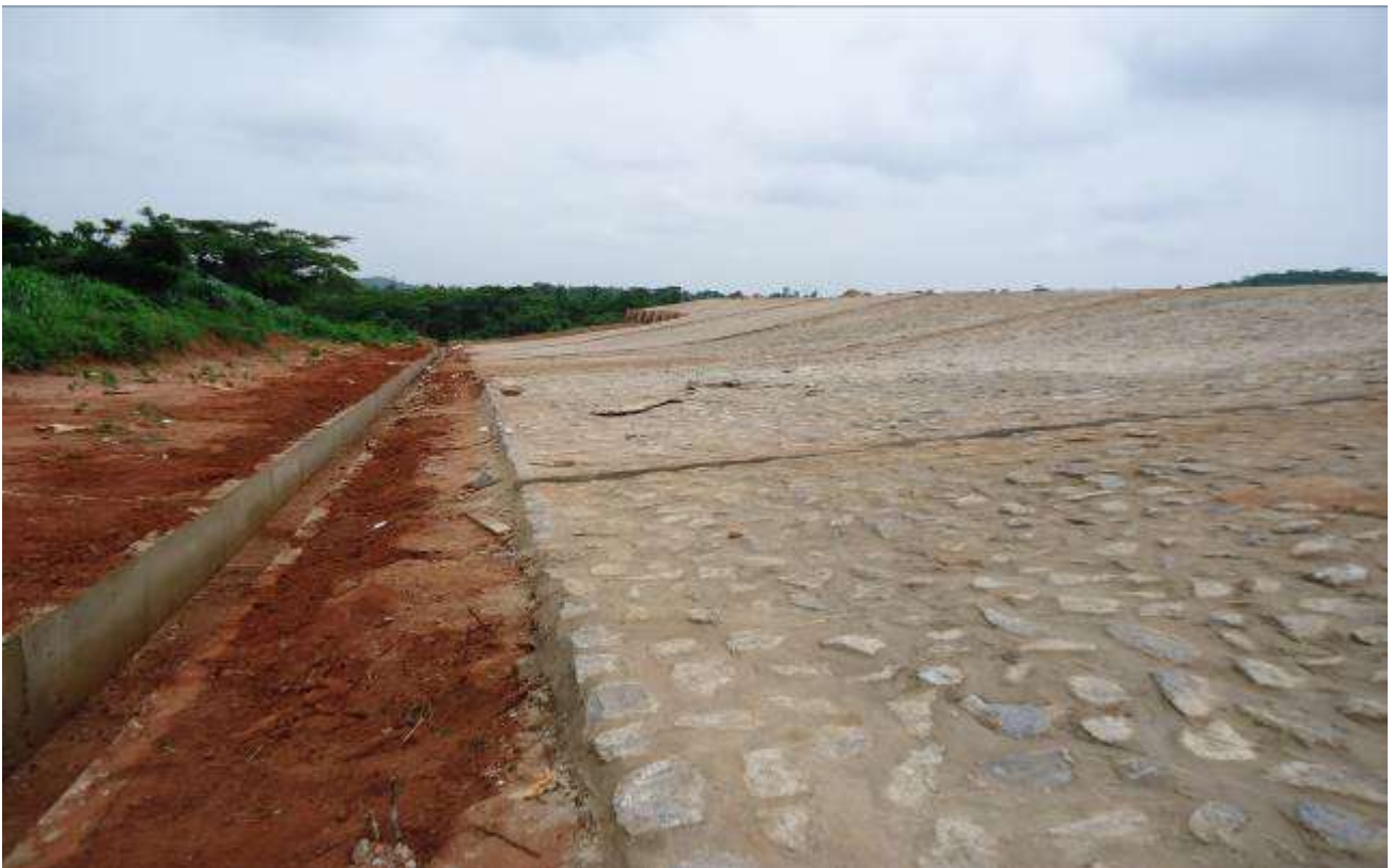
Retaining wall and drainages at New Abeokuta Sub-station by - By Lumkalt Energy Limited . Note: Stone pitching works not inclusive.
