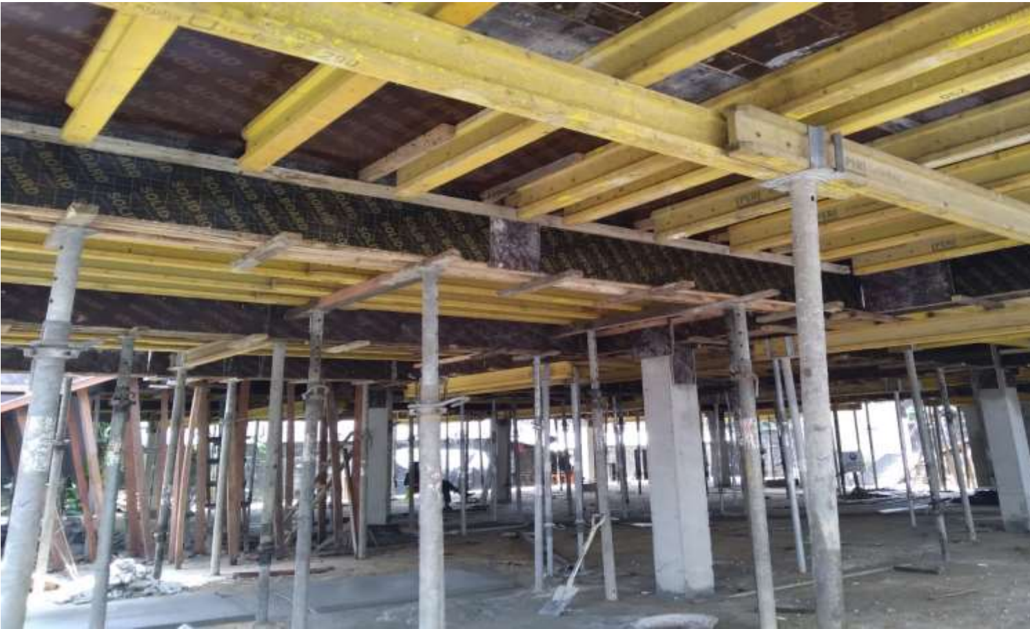
formwork on first floor beams and slab Completed
