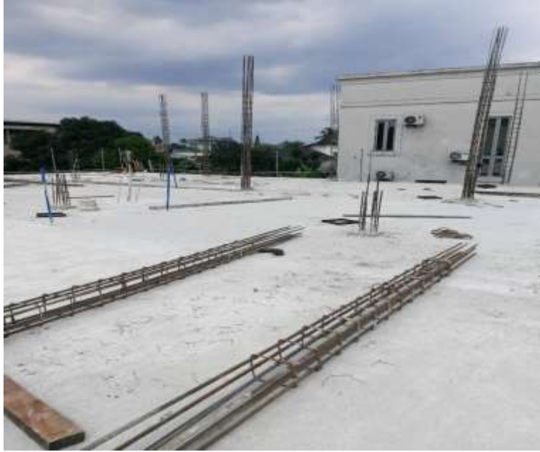
Placement of First Floor to Second Floor Column Reinforcement Ongoing
