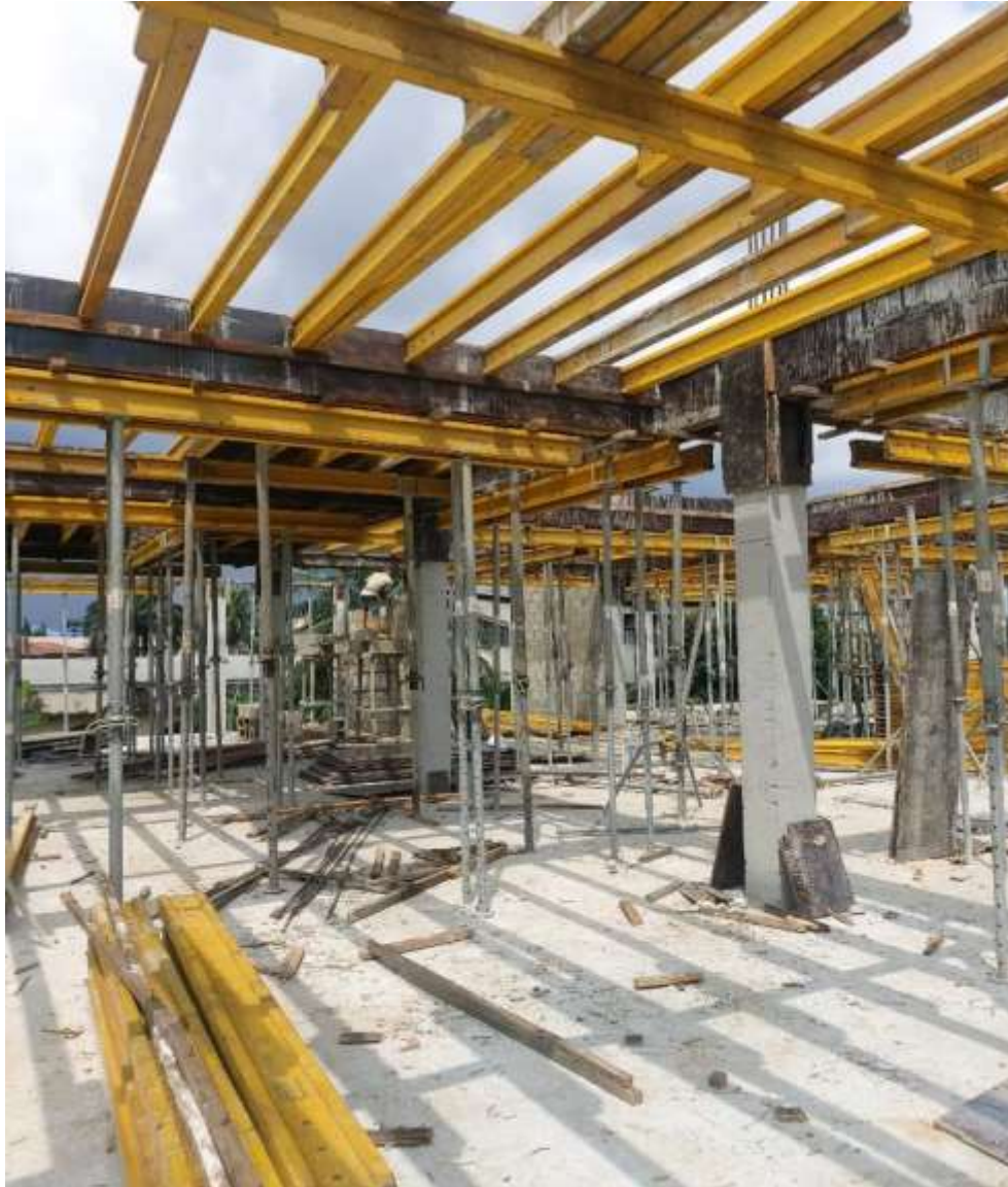
Placement of second floor beam and slab formwork Ongoing
