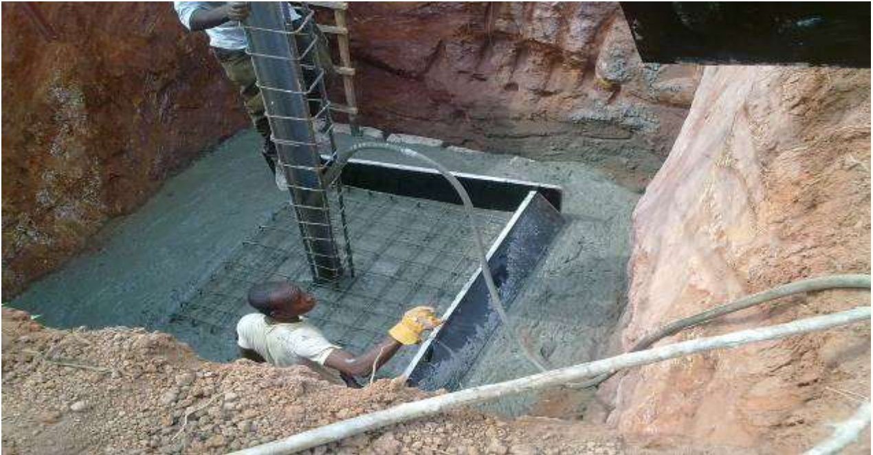
Construction of formwork and footing pad (New Abeokuta to Papalanto) - by Lumkalt Energy Limited
