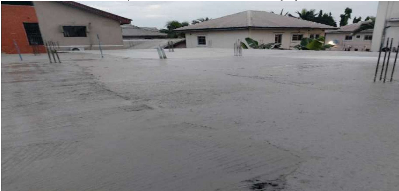
Concrete placement of the first floor slab and beam ongoing
